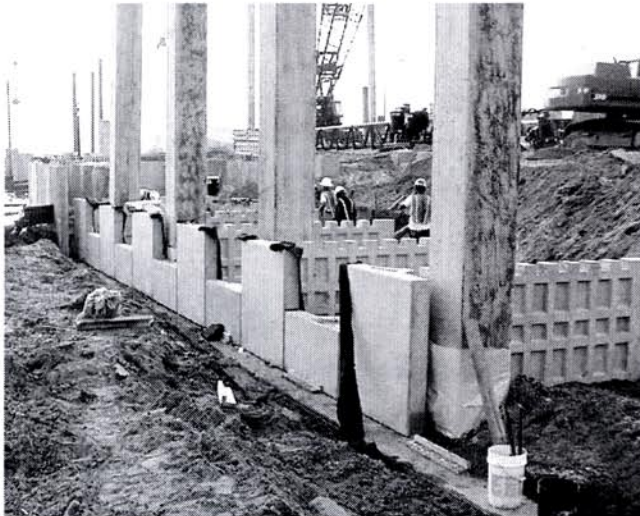
Hathaway Bridge, Panama City, FL
