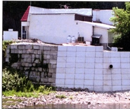
Embankment Repair – Ice Scour Montpelier, VT
