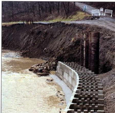
Bank Stabilization - Flood Wegee Creek – Shadyside, OH
