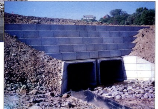
Terraced T-WALL for Barrington Manor Warrendale, PA
