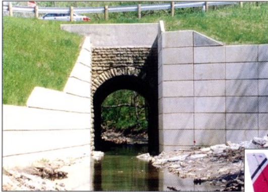
T-WALL with existing stone culvert Hamilton County, OH
