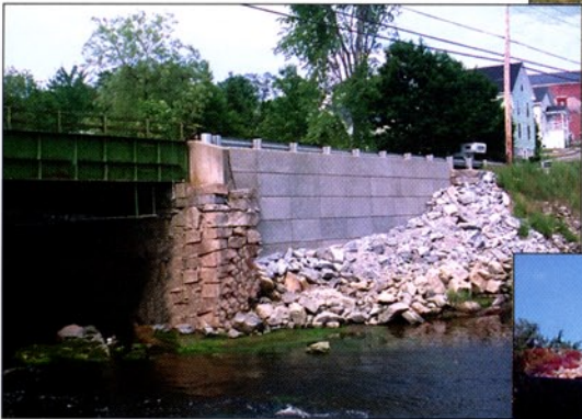
Maine DOT Bridge Rehabilitation Waldoboro, ME
