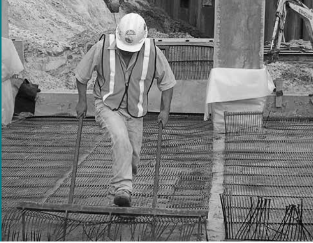
IMAGE O: Uniaxial geogrid shall be tensioned prior to fill placement.
