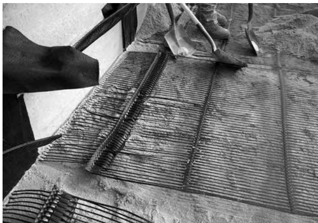
IMAGE S: Bodkin connection used to connect geogrid panels to geogrid tab.
