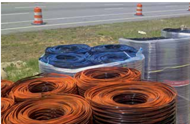
IMAGE C: Color coding of geogrid panels allows for quick, accurate identification even after labels are removed.
