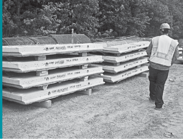
IMAGE A: ARES® panels should be stacked on a level, stable surface provided by the Contractor. Dunnage shall be carefully selected to allow panel separation and placed to avoid panel cracking.
