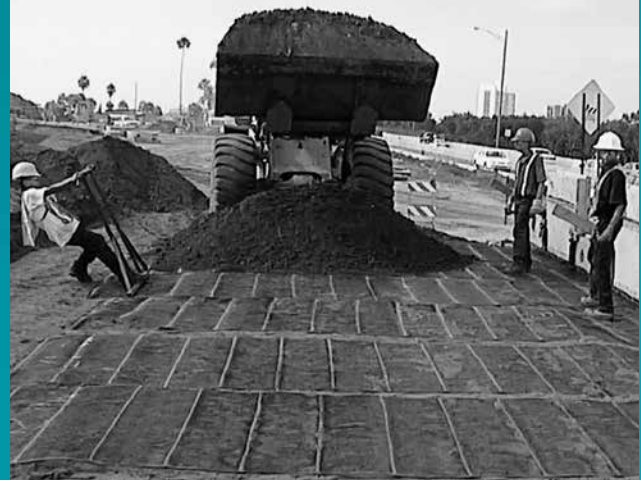
IMAGE P: Placement of fill on tensioned geogrid.
