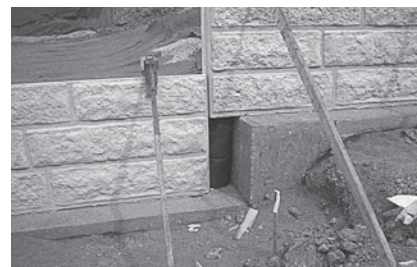
IMAGE G: Upper leveling pad offset 9 in.
