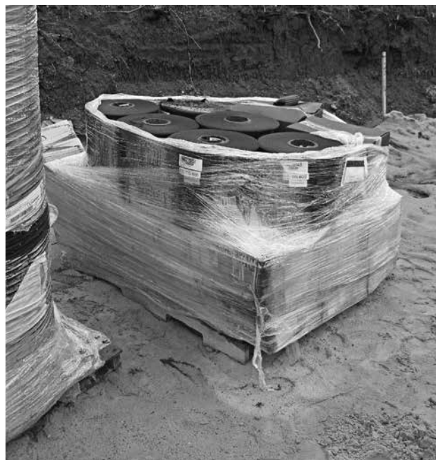
Palletized component materials upon arrival at site.
